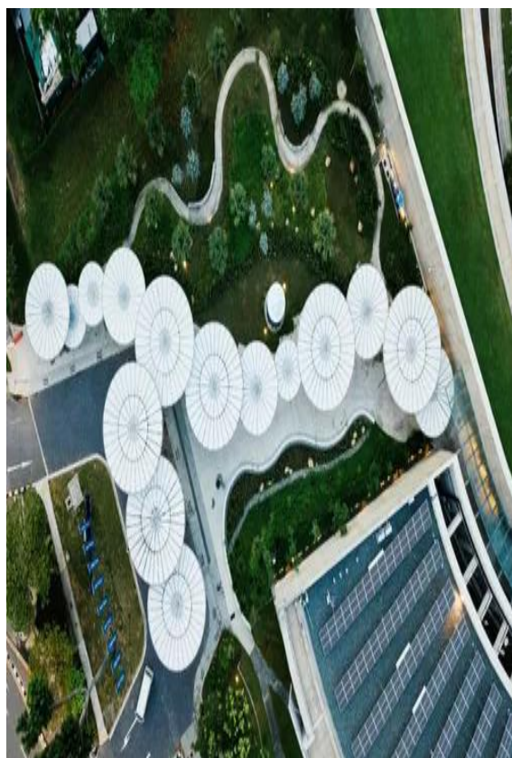
Fig 1. Using of solar plants on the rooftop
